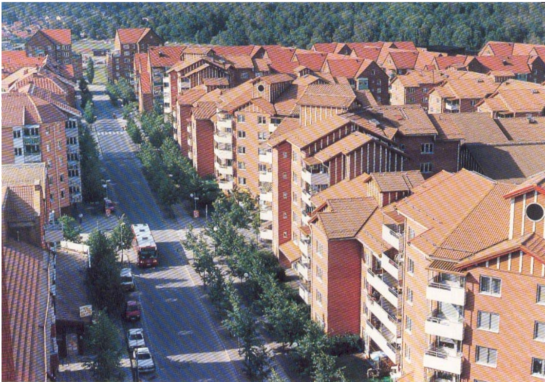
Picture 1: The Avenue in Skarpnäck.
